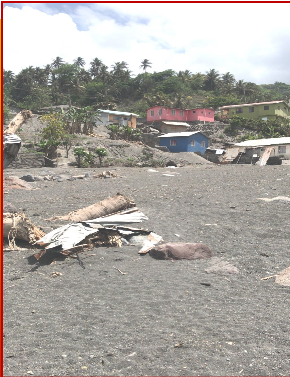
Damage to a building in the Red Zone.
