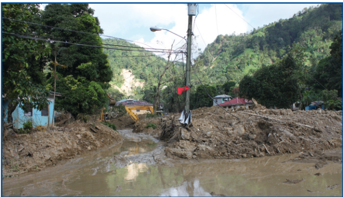
Hurricane Tomas damage
